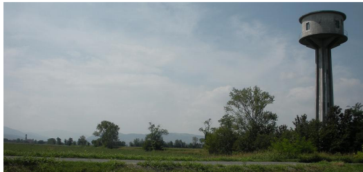
Figure 4: South view from the site
